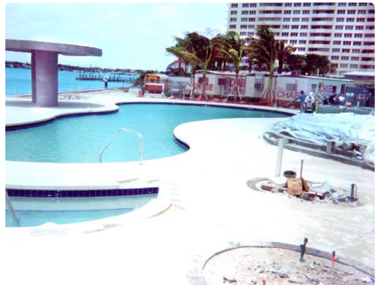
Pool and Deck Area Under Construction
