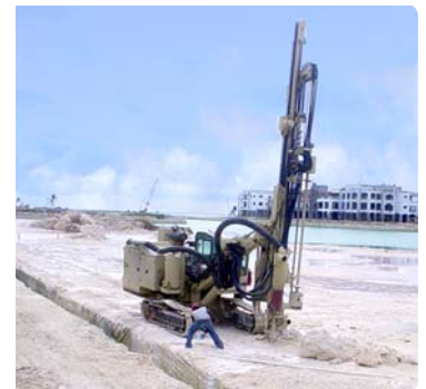
Construction in Progress
